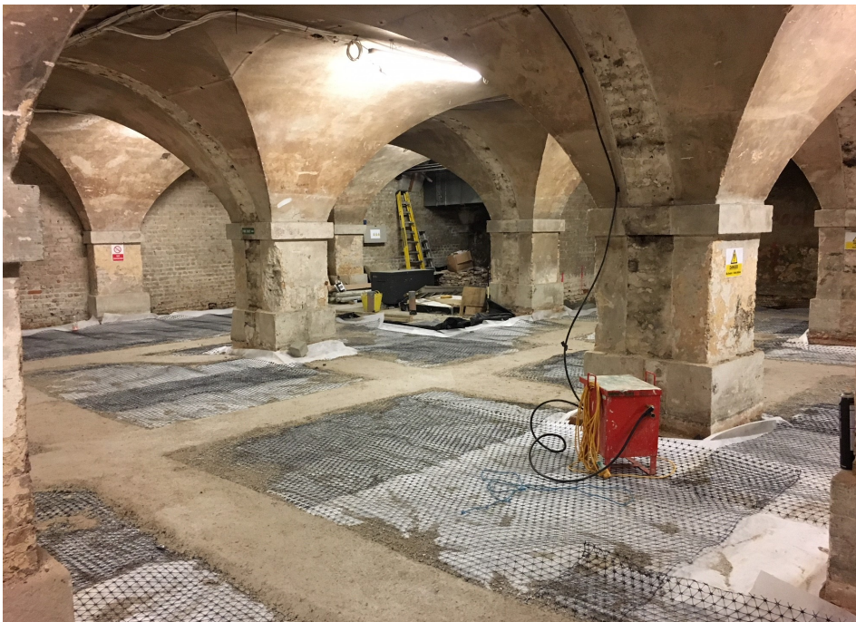
St George's Undercroft: a new floor is laid.
